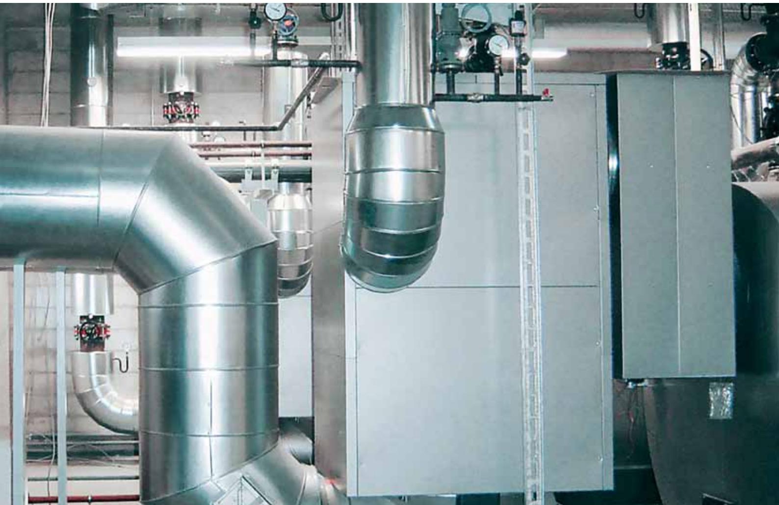
Downstream Vitotrans heat exchanger fitted to a Vitomax boiler
