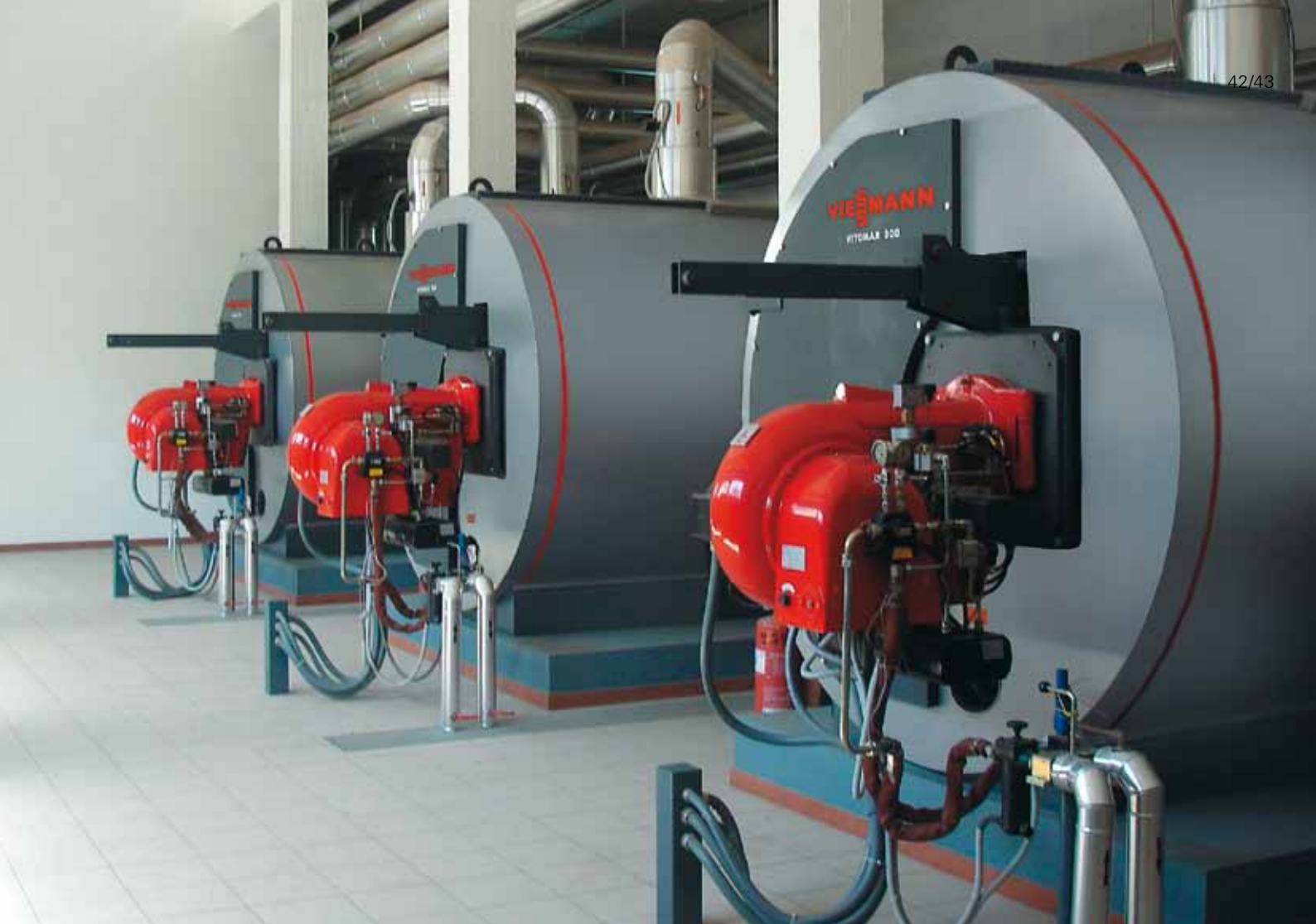
Vitomax 300-LT low temperature hot water boiler
