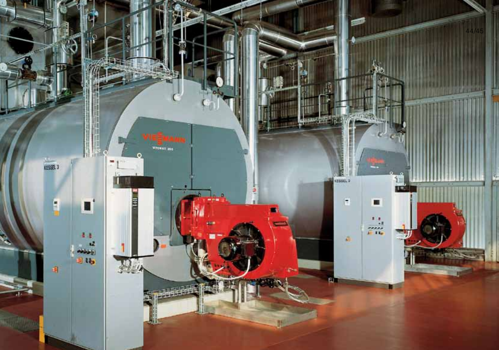
Vitomax 200-HW high pressure hot water boiler
